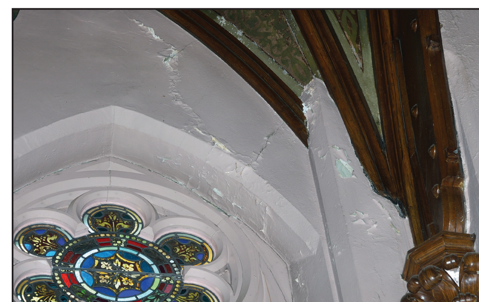
Water damage in the Organ Loft
