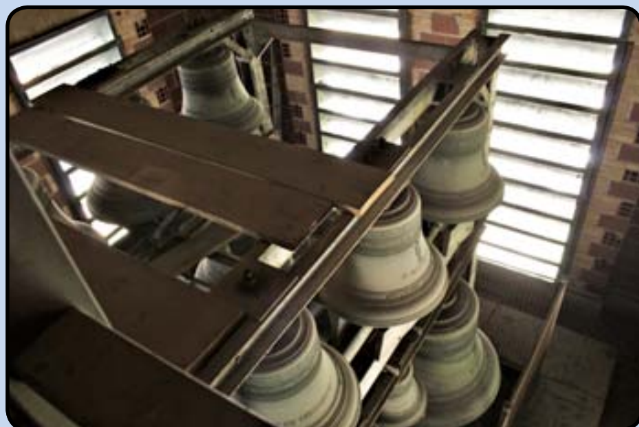
Twelve bells are securely suspended in the east tower from steel beams.
