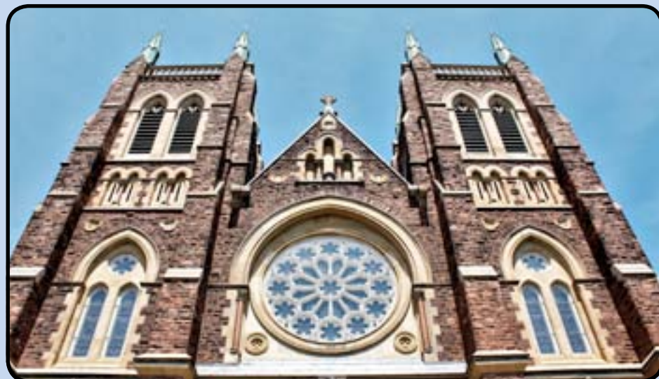
This photo shows the two slightly different colours of Medina sandstone in the Cathedral towers.
